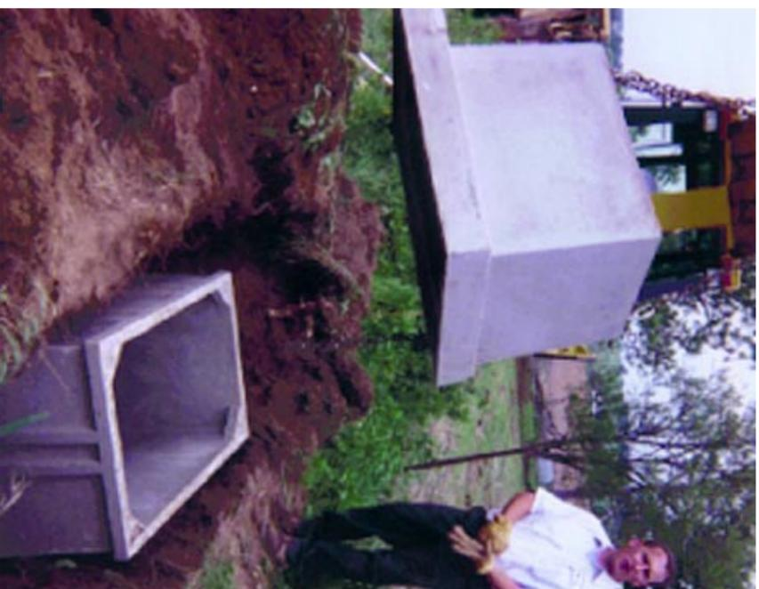
2. Set the base. Bases are available as grade-level flat slabs, or with integrated riser sections to elevate the equipment, providing protection from snow, surface water, grass fire, and to make servicing the cabinet more convenient.
